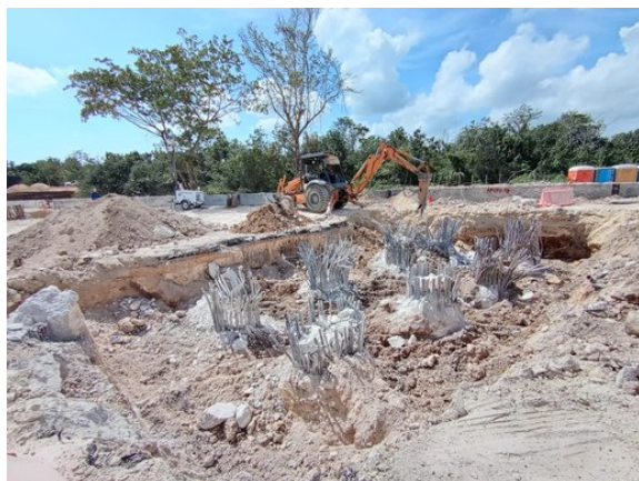
Earthmoving at the work front.
