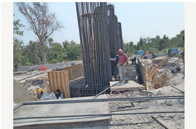
Formwork for foundation elements.
